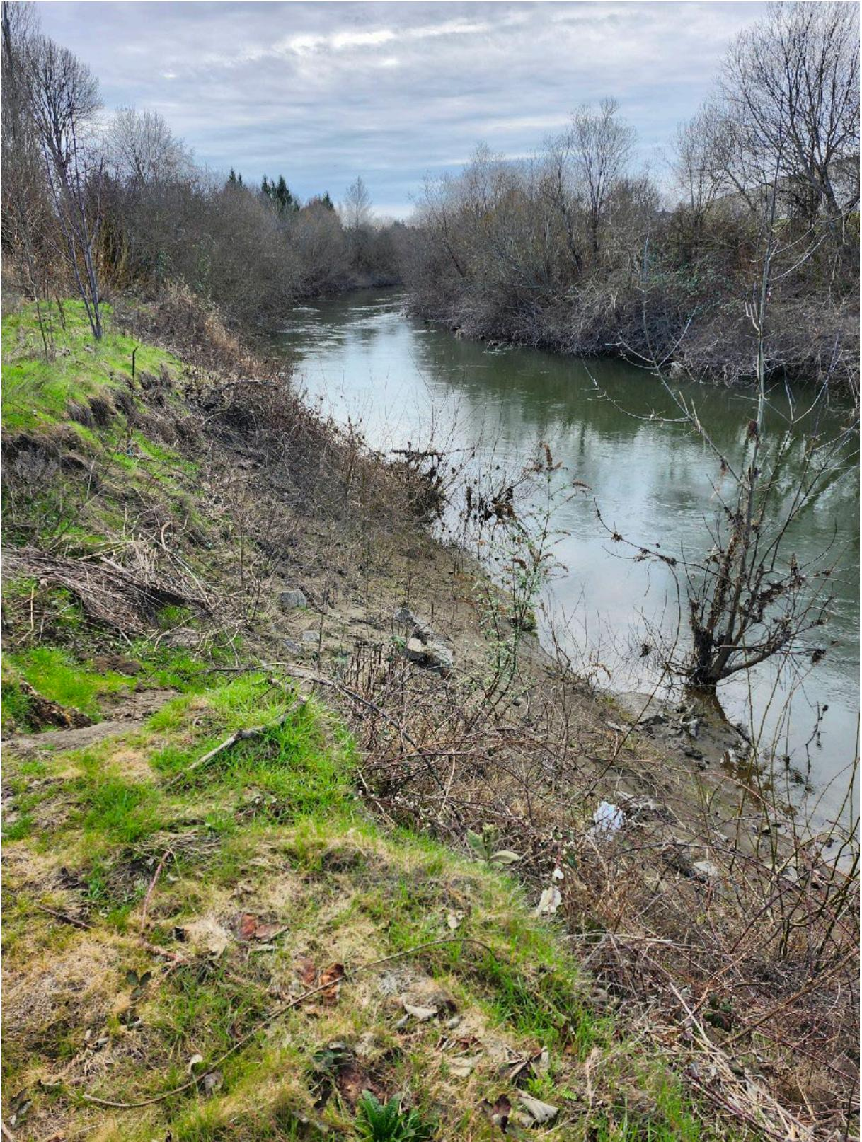
Photo A-5. Erosion of riverward levee face. Scattered riprap over mixed earth. Upstream orientation. Approximately RM 15.15.
